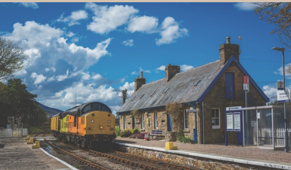
Class 37 with track testing train passing through Forsinard Station.
