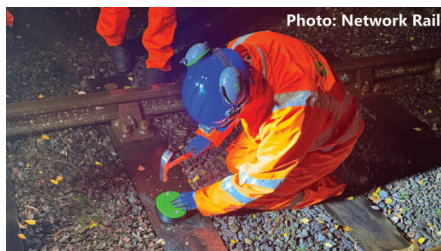
Installation of beacons is simple and quick
